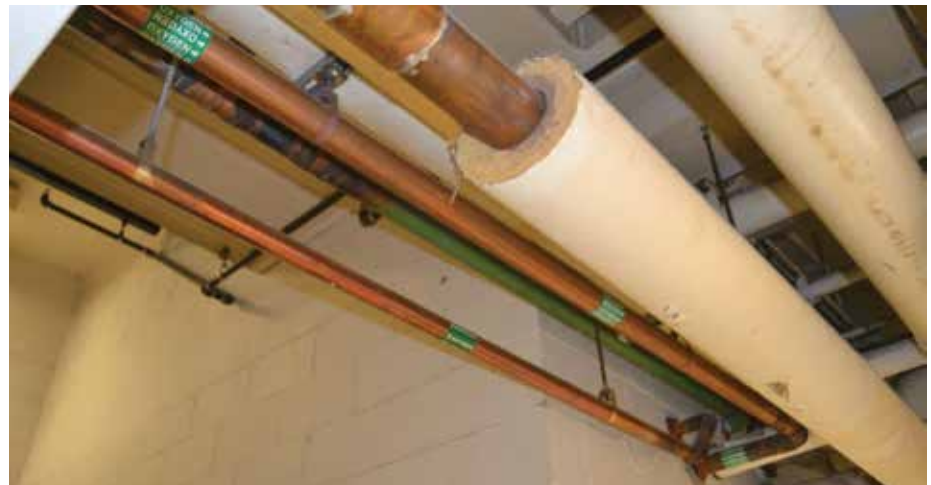
Figure 3: Pipe not completely insulated
